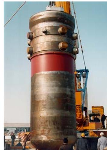
The most important ageing effect on the RPV in a nuclear power plant is embrittlement. Embrittlement leads to the reduction of toughness of the materials and thus to a higher risk of vessel failure.
