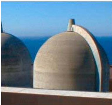
The containment is a large steel building, usually with a hemispherical dome. Containments are often not visible since they are usually surrounded by a steel or concrete building that provides additional boundaries and aesthetically pleasing designs.
