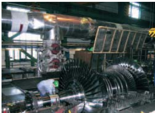
picture 2: Working at the turbine of DUKOVANY unit 3
